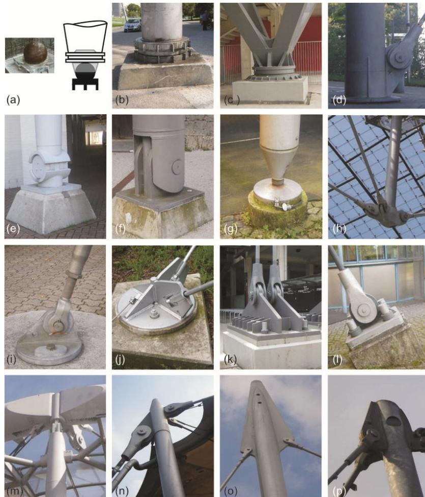
(a, b, c, d, e, f, g) base (with ball joint) of hinged masts; (h) base of flying mast; (i, j, k, l) base of cables; (m, n, o, p) components anchor points on the top of the masts. Image (a): mast ball joint later cast in concrete) by SCHLAICH (2003), p.109; images (b-p) and sketch (a) by author.
