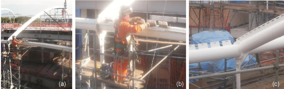
(a, b, c) welding of new row of plates at internal ring
