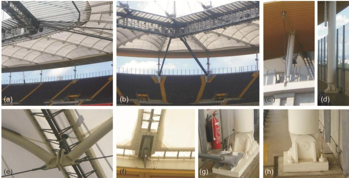
(a) views: internal, external; (b) corner of the polygon connected to the bleacher concrete structure by tubular profiles (c) masts and pre-tension cables; (d, g, h) mast details; (e) aches with pre-tension cables; (f) joint between saddle shape modules; (images by author).
