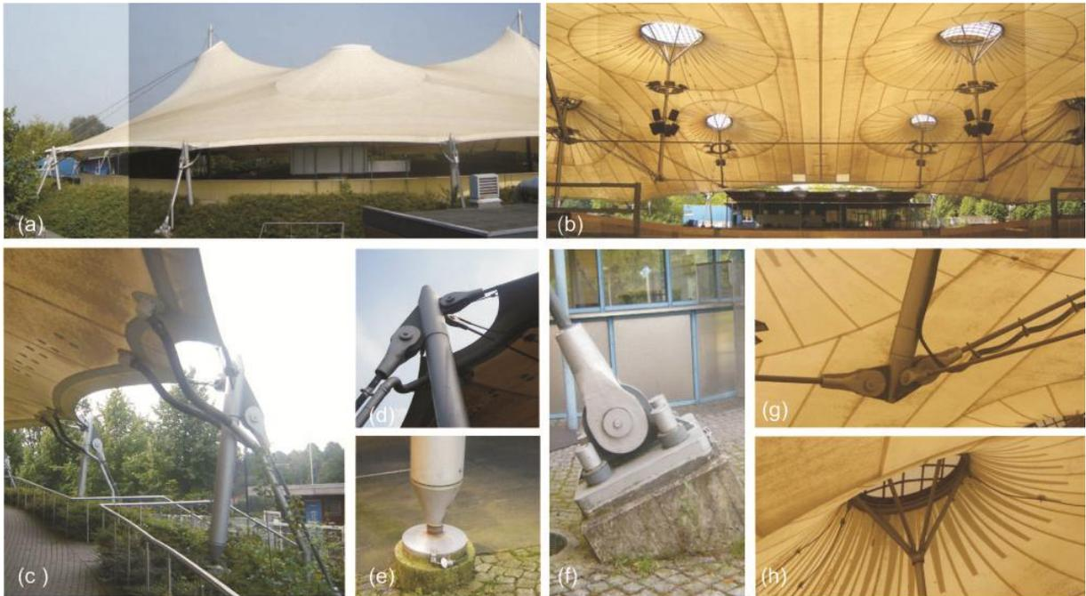
(a, b) external and internal views; (c, d, e) top and bottom of small masts (f) cable anchors, (g,h) top and bottom of flying mast; (photos by author).
