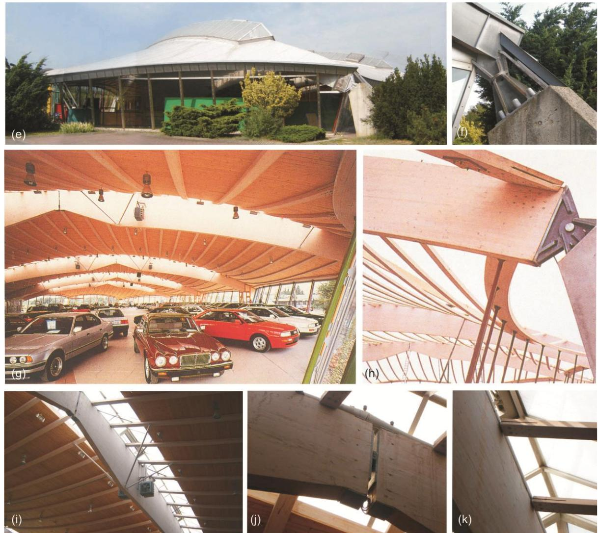
(a, b, c) 3D view, plan and vertical section syst. support; (d- det1, h)) anchoring of the three-hinged arch; (d- det2, f) points of pre-tension of the edge arch; (e) external side view; (g) internal view; (i) overhead lighting on three-hinged arch, (j, k) three-hinged arch and purlins; (f, i, j, k) images by author; (g, h) photos: Friedhelm Thomas, Krefeld (*Informationsdienst Hols*, 1996); (a, b, c) sketches by author; (d1 e d2) drawings by Prof Dr Baier.
