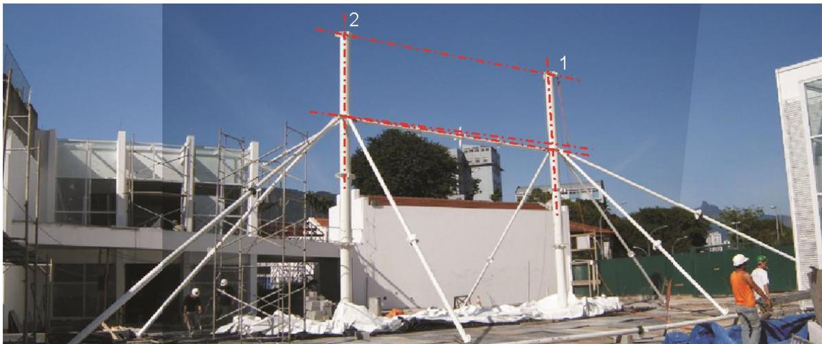
Mast inaccuracy: profile connections in different levels
