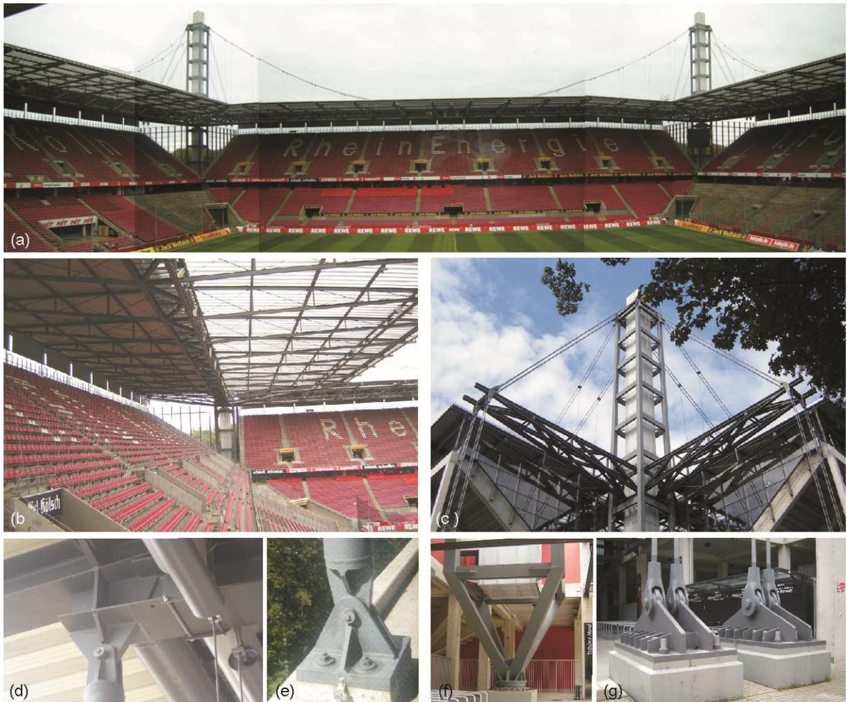
(a) internal view; (b) roof of the bleachers; (c) mast; (d,e) detail of tubular profiles; (f, g) anchors of the mast and cables (images by author).
