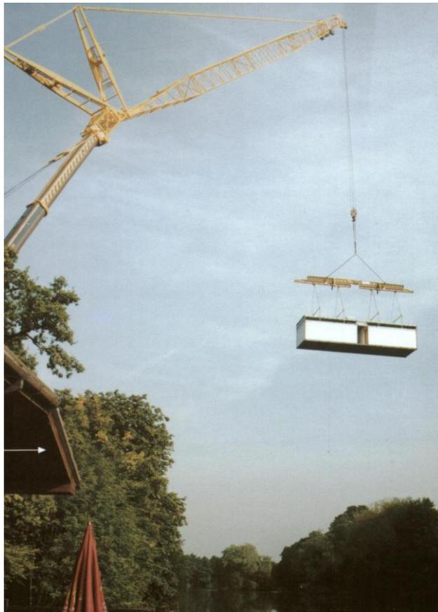
Figura 6.9: Sistema de transporte vertical (THE ARCHITECTS' JOURNAL, 1999, p. 30)
