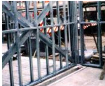
Figura 4.7 – Grade estrutural instalada (SCI, 1994, p. 26)
