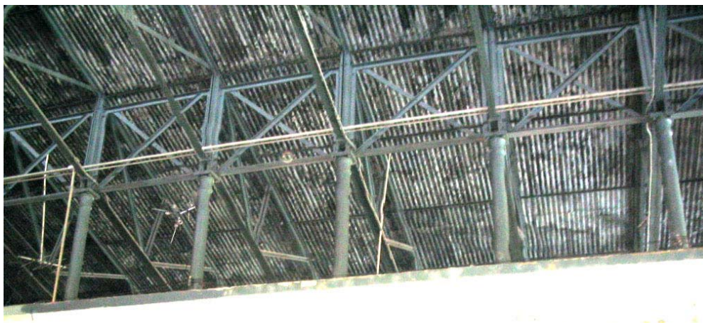
(c) Vista interna, mostrando as colunas e as vigas treliçadas.
